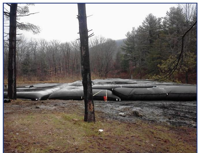
The Geotube® containers were filled with the chemically conditioned sediment and were left to consolidate before they were excavated.
