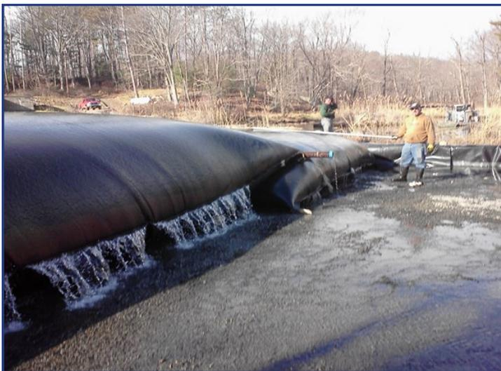
Clear filtrate is released from the Geotube® containers.
