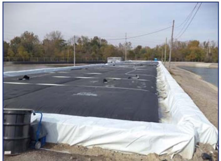
The Geotube® containers are beginning to fill up in the containment pad which has a 15-mL liner to contain and direct the water back to an adjacent pond.
