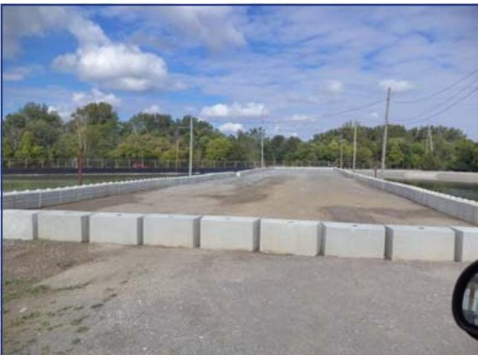
WaterSolve provided a drawing for this containment pad and a contractor graded it per the drawing. Jersey barriers were placed around the perimeter as a containment wall for water and the Geotube® containers.
