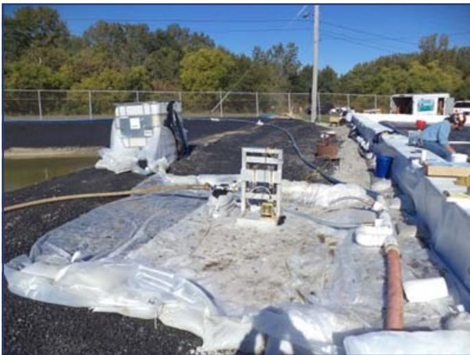
The polymer make-down unit is placed adjacent to the Geotube® containment and it injects the Solve 216B into the residual pipeline.
