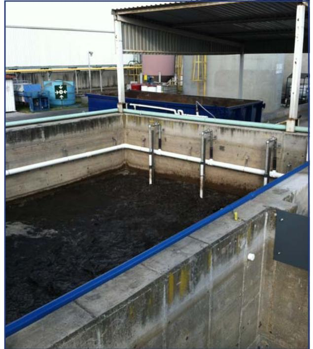
Aerobic digester sludge will be dewatered in an MDS container placed in the dumpster box in the background.
