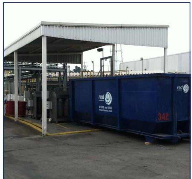
The MDS will be placed in the dumpster. Released filtrate will flow to an existing floor drain located where the yellow curbs meet.
