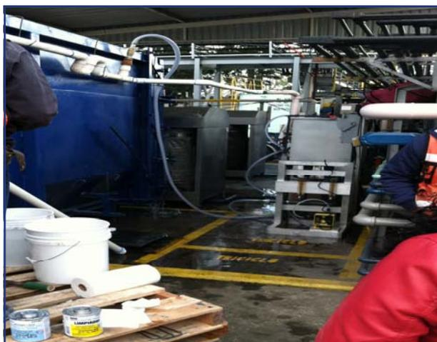
The polymer make-down unit is activating the polymer and injecting it prior to the elevated white mixing manifold. The treated material is then deposited into the MDS container.
