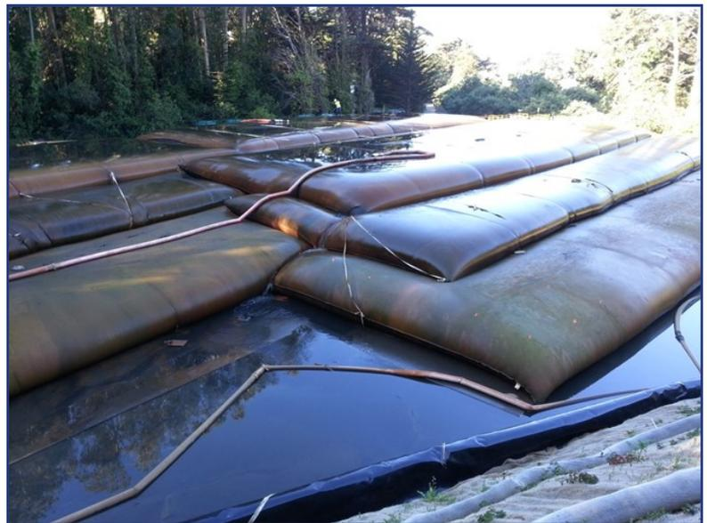
Due to space limitations, three layers of Geotube® containers were stacked in the material handling area.
