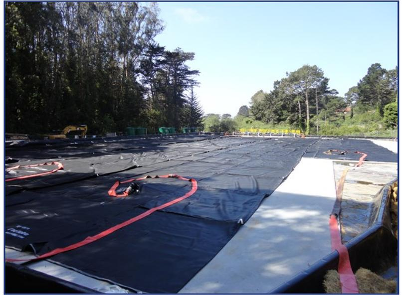
The first layer of Geotube® containers was deployed and connected to the dredge pipe.
