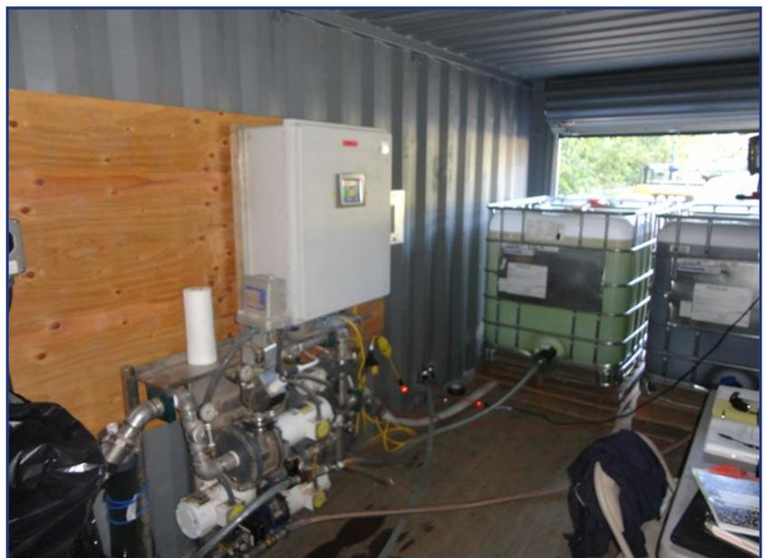
WaterSolve's CCTS (Chemical Control and Tracking System) was installed in a conex box along with the coagulant and flocculent.
