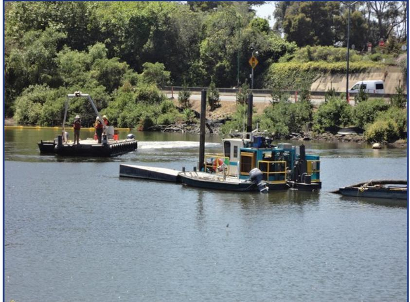
This hydraulic dredge dug the material from the lake and transferred it through an 8" HDPE pipeline to the Geotube® containers in the material handling area.
