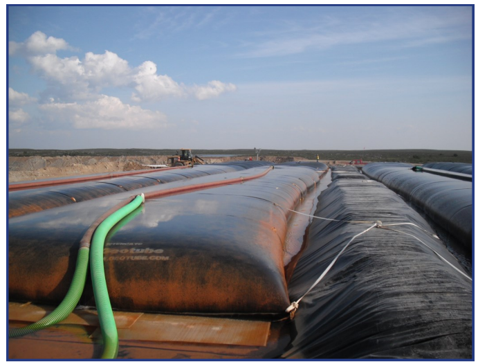
The Geotube® containers under full scale operation.
