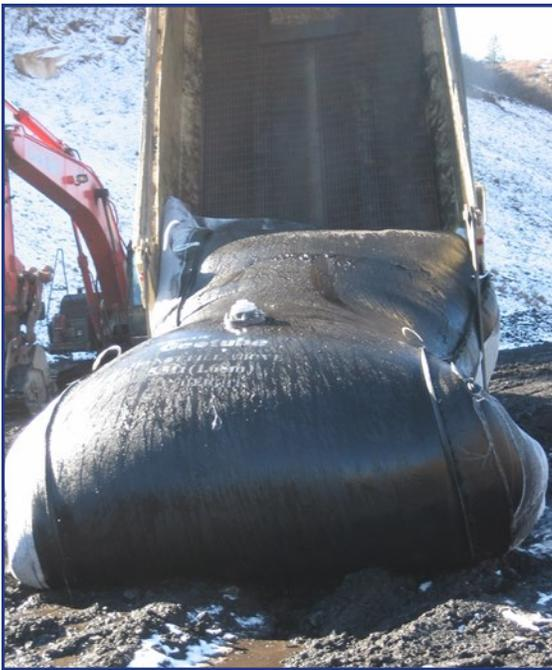
The first Geotube® container is dumped at the disposal site (left).
