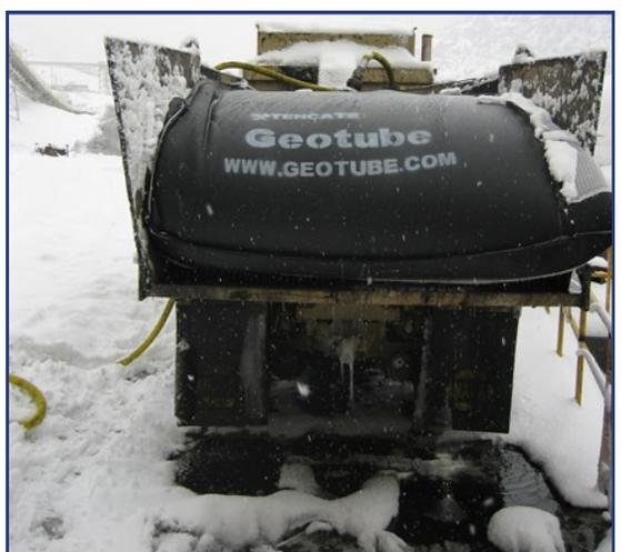
Plywood was added to keep the corners of the container from the potential pinch point of the tailgate support (right).
