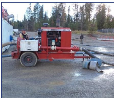
A 6" diesel pump transferred the biosolids from the frac tank on the left to the manifold near the Geotubes via a 6" pipeline. The pump has a flow meter and a valve to limit the flow if needed.
