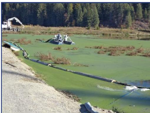
This 50-hp electric dredge sent the biosolids to a frac tank where they screened for debris and mixed.
