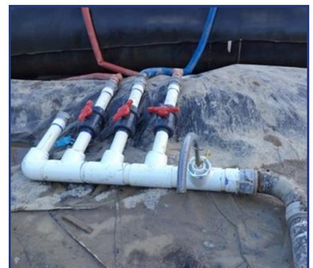
The 6" hose connects to a manifold with a sample port and a series of 4" laterals that can be directed to fill ports on the Geotube® containers.
