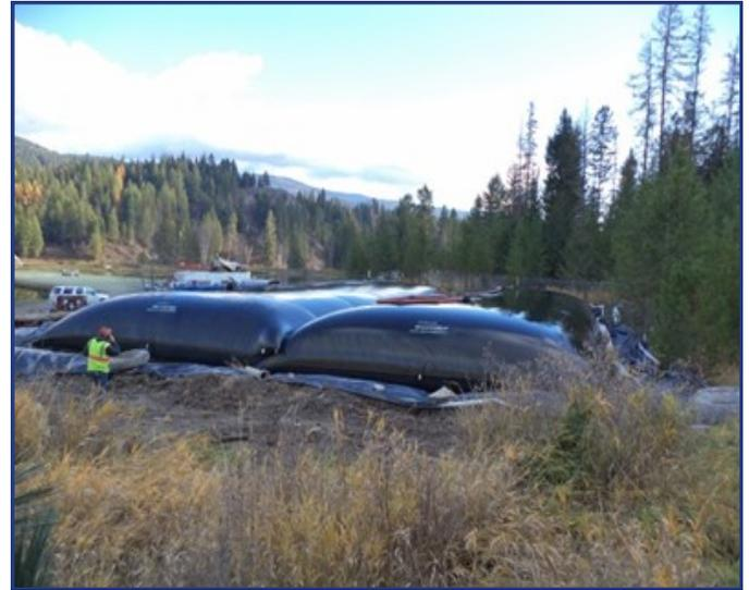
Two 70' circumference by 100' long Geotube® containers were placed in containment to capture and dewater the biosolids at this Washington wastewater treatment facility.
