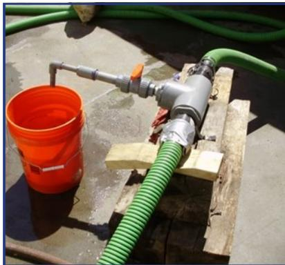
This inline sample port allows visual observation of the polymer dose to determine if the feed rate needs to be adjusted.
