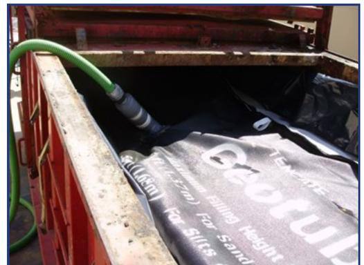
The 2" pipeline is plumbed into the fill-port of the MDS Geotube® which is inside the 30 cubic yard roll-off container.
