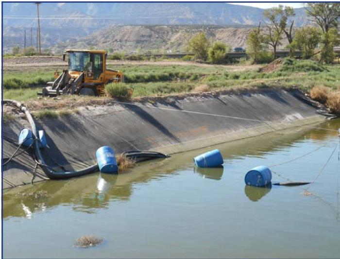
Biosolids lagoon during early stage of the project. A 6" submersible pump was suspended on a cable and the material was pumped to the Geotube® containers.
