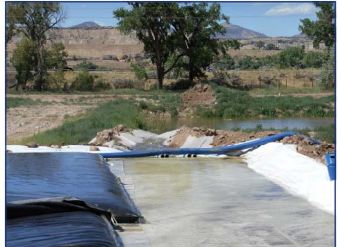
As the Geotube® containers begin to fill, the filtrate can be seen releasing through the pores of the GT500 material. The laydown area was graded to direct the filtrate to a holding area adjoining the low spot. By designing the site to utilize gravity flow for the filtrate, the cost of a filtrate return pump can be avoided.
