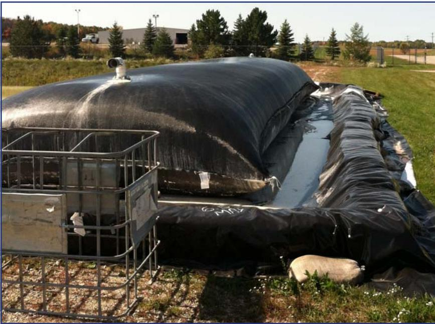
After a few weeks, the Geotube® container reached its maximum capacity. The hoses were disconnected and the City decided to let the container continue to dewater over the next several months.
