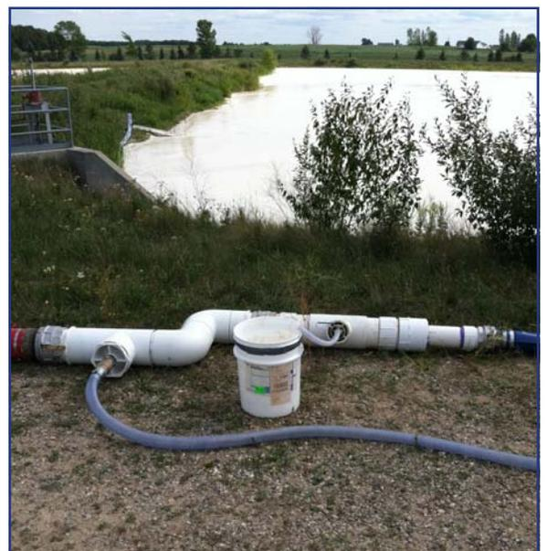
**(RIGHT)** Prior to the residuals being pumped into the Geotube® containers, Solve 163 was injected into the material to facilitate the dewatering process. Two ninety degree bends provide mixing energy so the chemistry and pumped material have adequate mixing.
