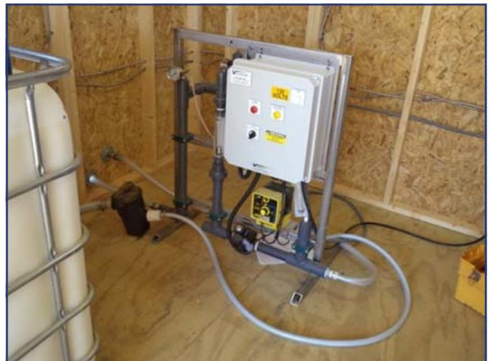
A Polymer Make-down Unit is used to activate the Solve 153 polymer and meter it into the 12" pipeline prior to the Geotube® containers.
