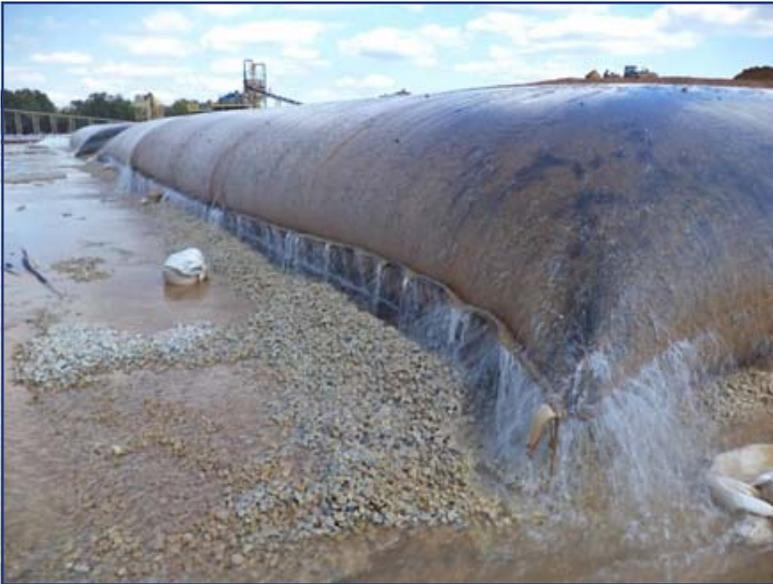
The Geotube® container is effectively capturing the solids and releasing clean filtrate water.
