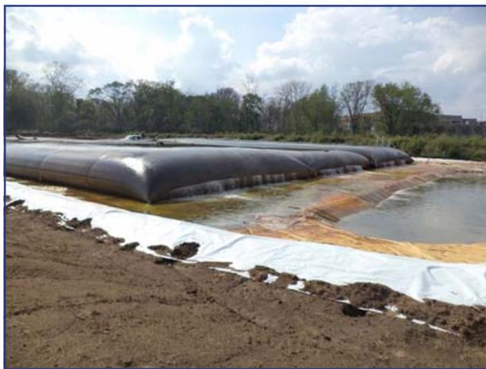
The Geotube® containers are dewatering very well in the containment area designed and drawn by WaterSolve's engineers.
