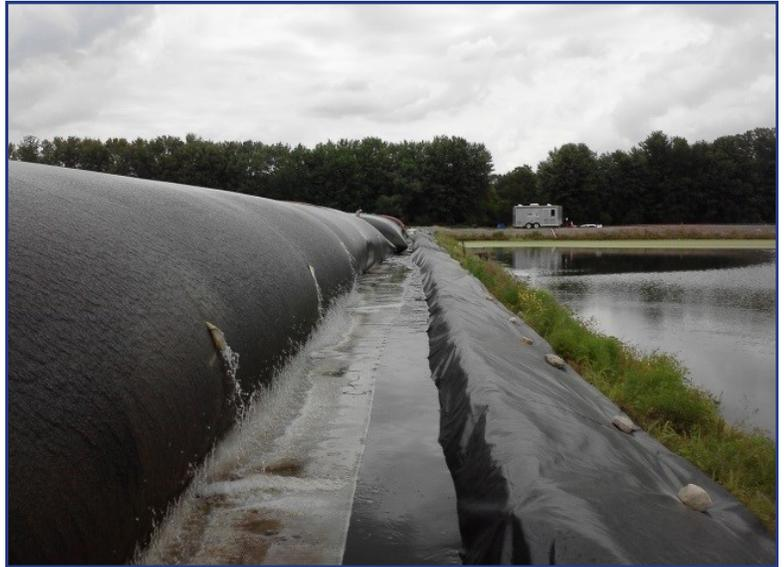
Clear filtrate exiting the Geotube® containers and is returned to the lagoon.
