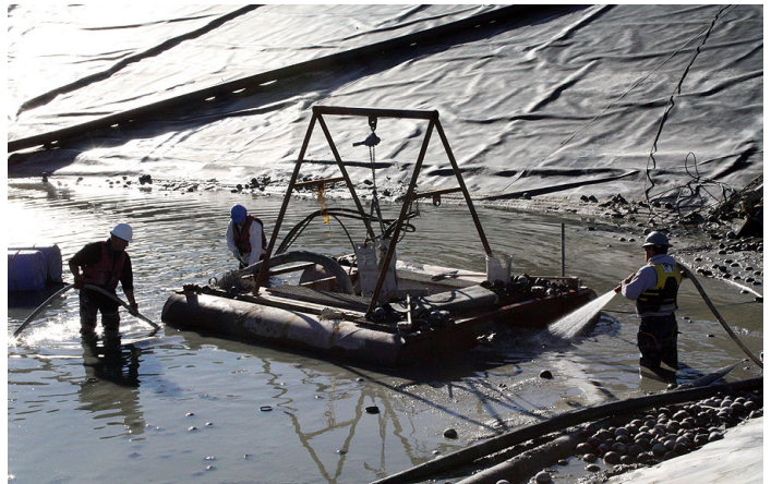
Pump required to overcome almost 500' of head was mounted on floats.
