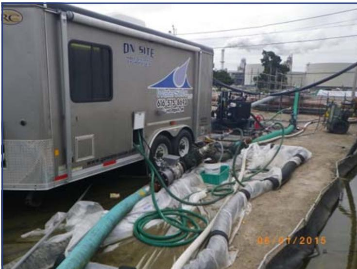
The Chemical Control and Tracking System (CCTS) trailer is parked along the 6" pipeline. The density and flow meters give information to the computer in the trailer and it automatically injects the proper dose of polymer into the pipeline.
