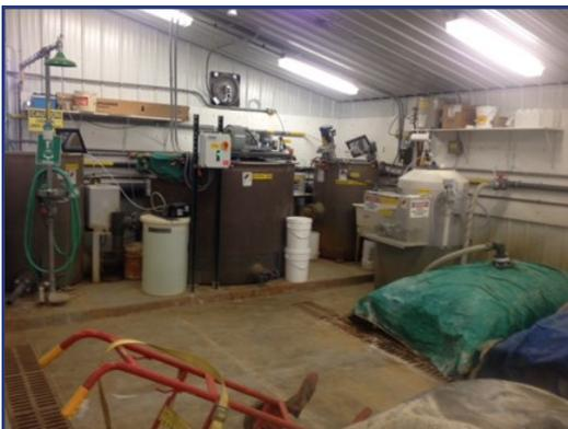
Left: Runoff water from the mining stockpile passes through this series of tubs as caustic, air, chlorine, and Solve 9244 are added to flocculate the solids.
