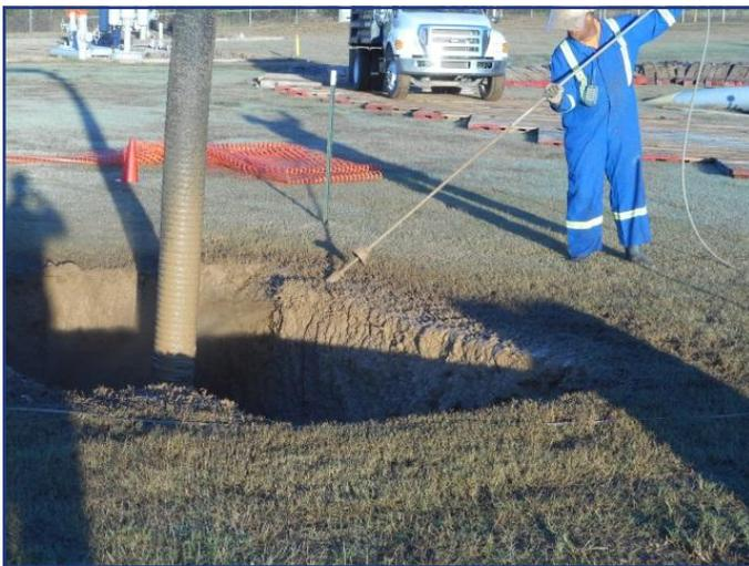
The hydro-excavating operator is using the high pressure wand to cut and slice the soil into the hole where it is sucked up by the truck.
