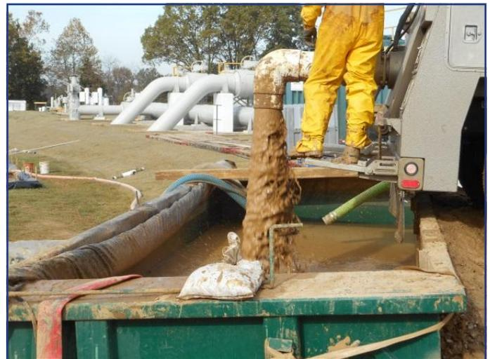
This 8" elbow directed the material into the dumpster with minimal splash. The pump is located at the far end. A lot of dilution was needed as some loads were really thick.
