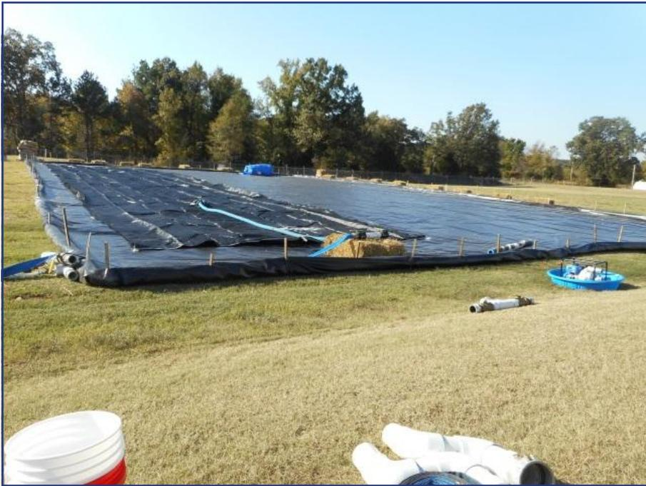
3 Geotube® containers were eventually filled in this containment area. The straw waddles had to be replaced with straw bales to provide more containment for the filtrate water.
