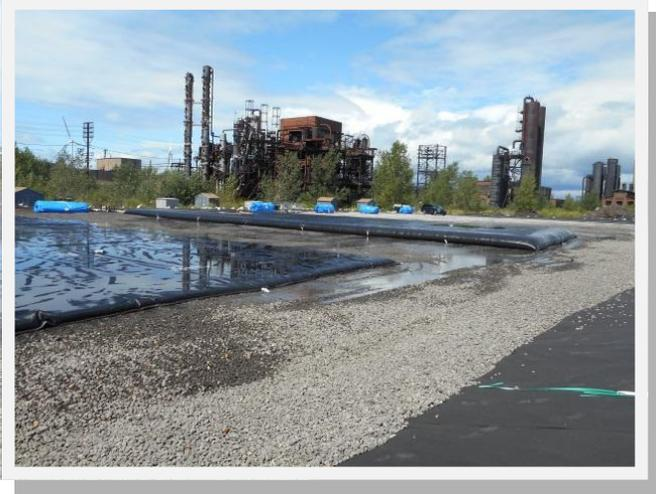
The Geotube® containers were placed on a bed of 1" gravel that is on a liner covered with felt. A 12" piping system returned the filtrate to the pits under the stone in the photo.
