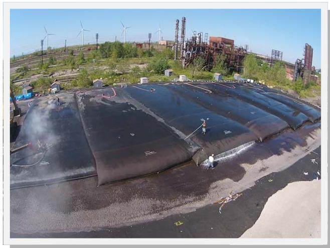
The material dewatered very well. It passed paint filter quickly. Cement is being added to the Geotube® container in the left of the photo to help stabilize the lead it contained before hauling it to a landfill. The tube in the center is being filled and is being smacked to help get water out quickly.
