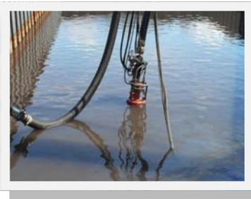
On left, the 6" hydraulic pump was attached to another excavator and is pulled through the water to suck up the material and pump it to the Geotube® containers.
