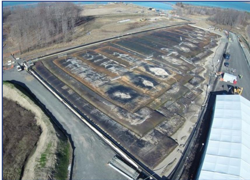
Over 5,000 lineal feet and three layers of 80' circumference Geotube® containers were used to dewater the contaminated sediment.
