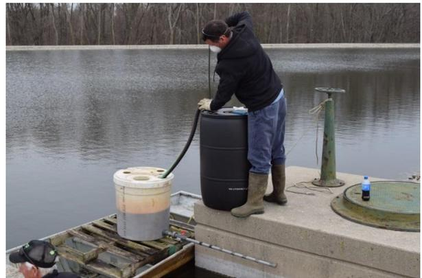
The Solve 3 is being pumped into the barrel on the boat which was placed on a pallet in the center of the boat. A pipe extends out over the boat and a valve controls the application.
