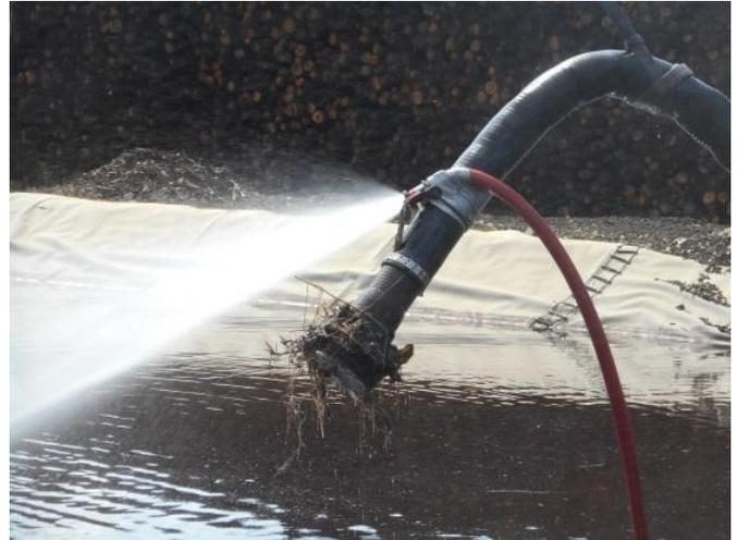
The suction hose is mounted on the cable held by a crane. The suction screen is full of debris. The fire hose is mounted to the suction hose to provide agitation and a steady flow of solids to the Geotube® containers. We learn new techniques on every job we do!!
