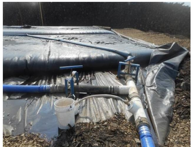
The sample port in this photo gives the operator a view of the effectiveness of the polymer and adjustments to the dose are made based on these samples. The pinch valves determine which tubes are being filled.
