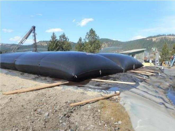
A pad was constructed on the bank of the pond which allows the filtrate to flow right back into the pond and no pumping is required.
