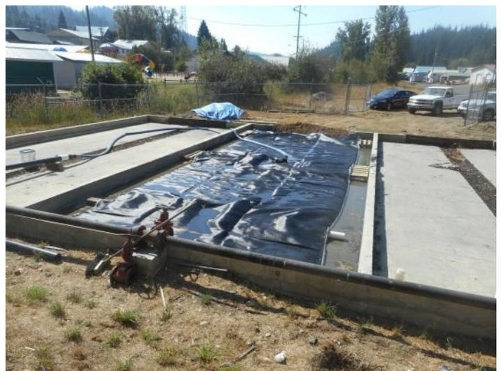
This Geotube® container fits very well in the middle drying bed. Some pallets were placed under the tube to allow better drainage and access into the sand in the center of the drying beds.
