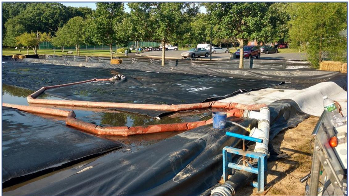
The polymer make-down unit and 6" manifold was set up near the lay-down area. A sample port was installed after the polymer injection to monitor the polymer treatment.
