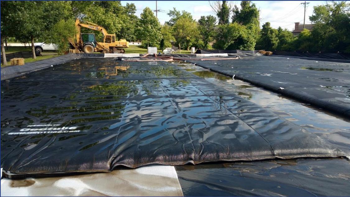
Two Geotube® containers were deployed and filled with lake sediment.
