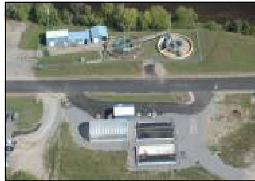
Award Winning Bonnechere Valley Township Geotube® Sludge Management Facility
