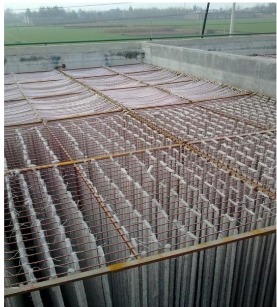
**Treatment Plant being upgraded with Biofilm Technology**
